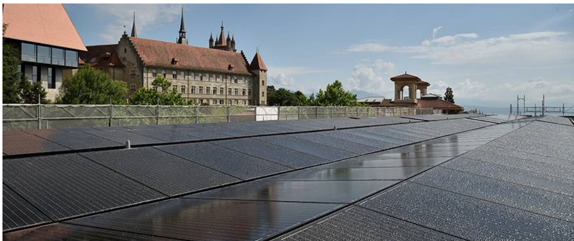
Figure 10. View of the photovoltaic roofing.
